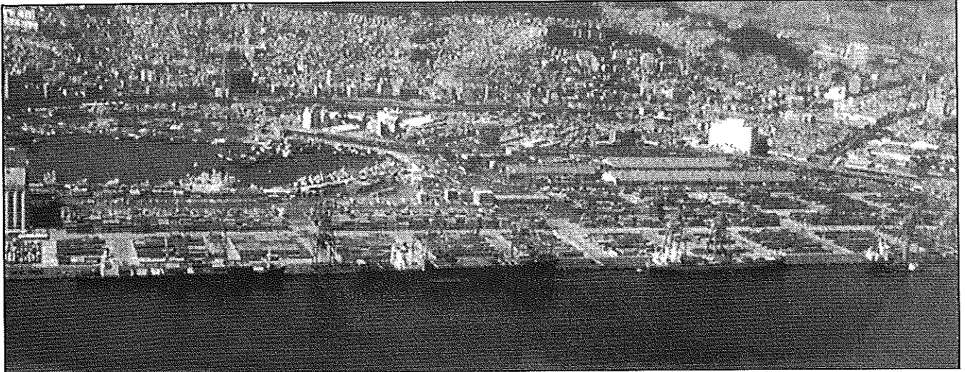
Pusan container terminal - "Vast industrial complexes have almost literally risen from the sea".
